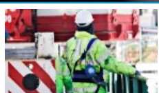
A day at the Atocha-Chamartin high-speed train worksite with FCC employees.
