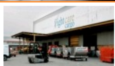
Visiting the air cargo area managed by Flightcare at Barajas Airport.
